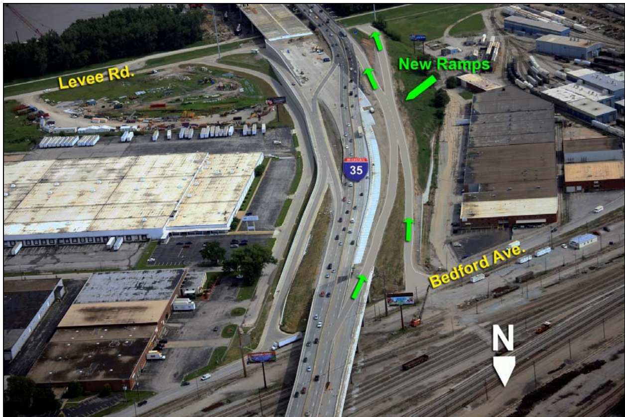
Enhanced Aerial View of the Levee/Bedford Collector-Distributor Ramp System on SB Interstate 29/35
