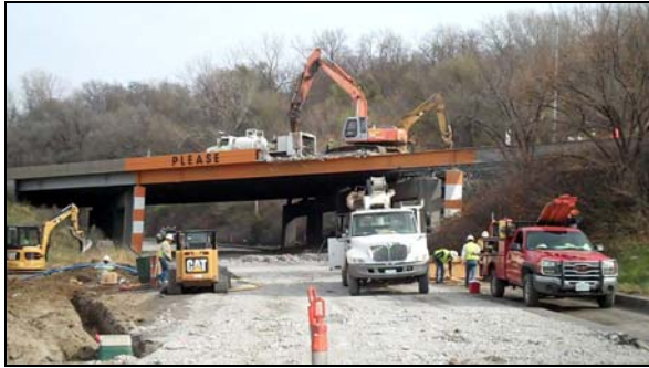
Paseo Bridge demolition taking place in November 2009.
