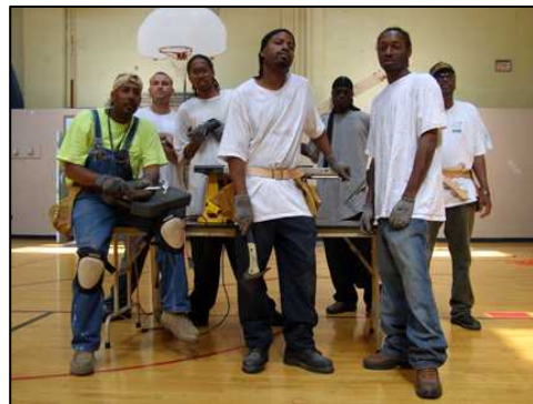
Helping repair bleachers at Nowlin Middle School as part of the Project Prepare program are from left to right: Brian Wilson, Jesse Jaschke, Kenny Lovelace, Dennis Jackson, Terrance Nelson, Ashton Shelby and Arthur Bailey.
